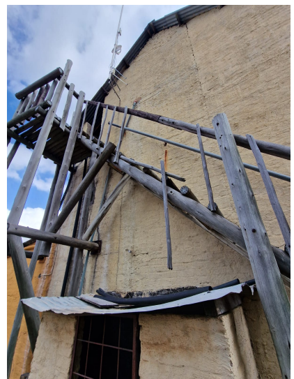
Staircase water tower
